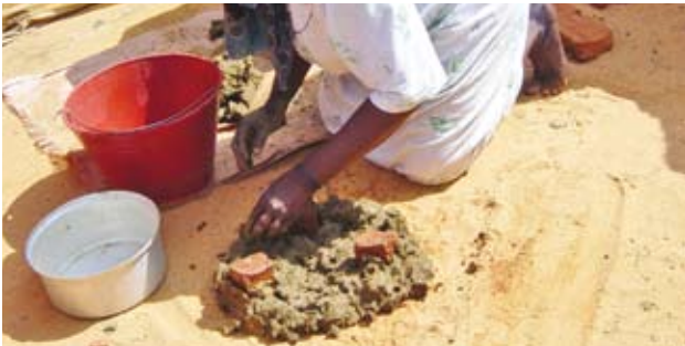
Pic 56. The whole circle is filled with clay to a depth of about 4cm.
