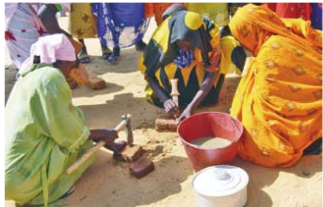
Pic 53. The red bricks are marked with a knife and cut into thirds using a small axe.
