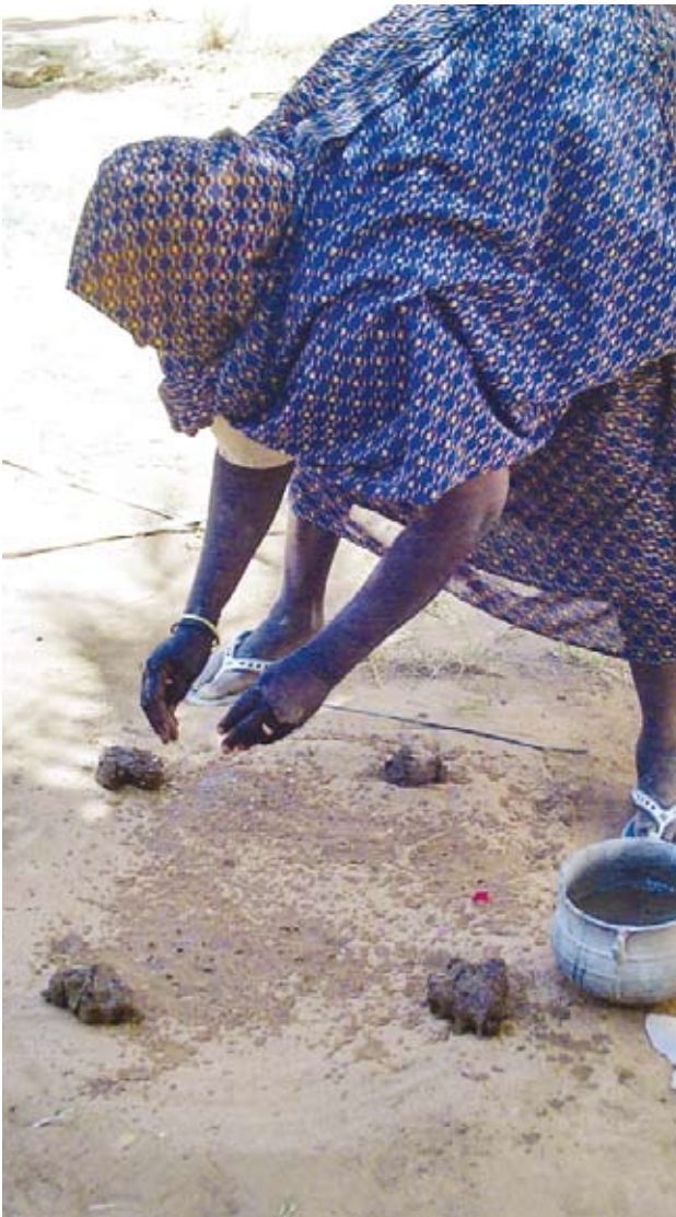
Pic 71. The size of the stove is marked out and clumps of clay mark its corners.
