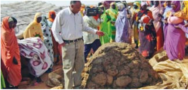
Pic 17. A completed pile of clay ready for use.
