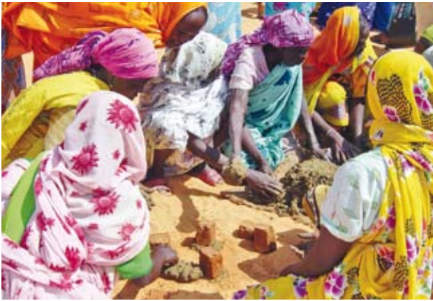
Pic 55. Three brick segments with clay stuck underneath them are placed an equal distance apart inside the edge of the circle drawn in the sand.
