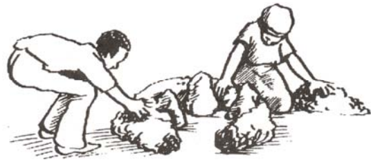
Figure 5.97 Smearing mud around the three stones
