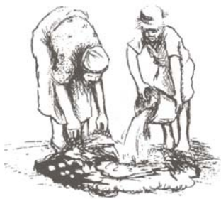
Figure 5.6 Mixing soil and water
