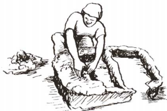
Figure 5.75 Building the top of the stove
