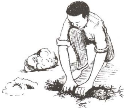
Figure 5.38 Rolling mud to form long pieces
