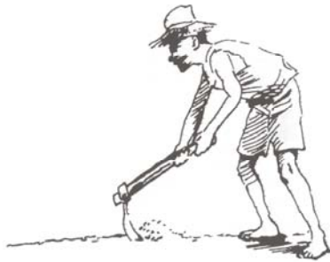
Figure 5.7 Levelling the ground
