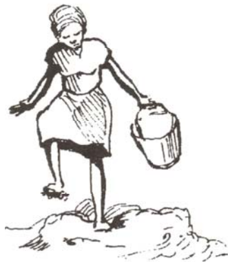
Figure 5.100 Mixing soil with water
