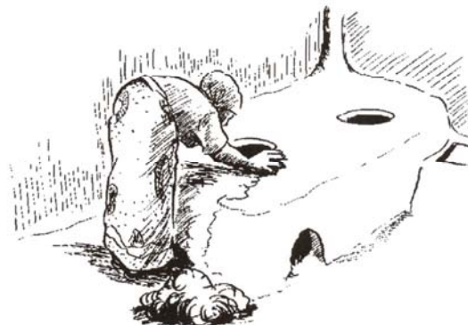
Figure A2.5 Filling in the crack
