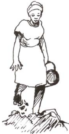
Figure 5.86 Mixing mud with water
