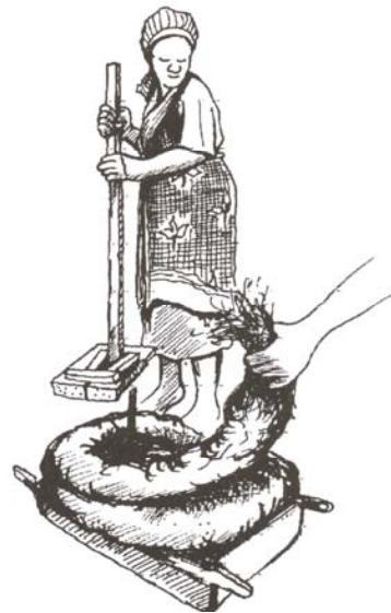
Figure 5.39 Compacting the mud rolls in the mould
