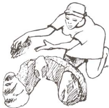
Figure 5.81 Smearing mud around the stones
