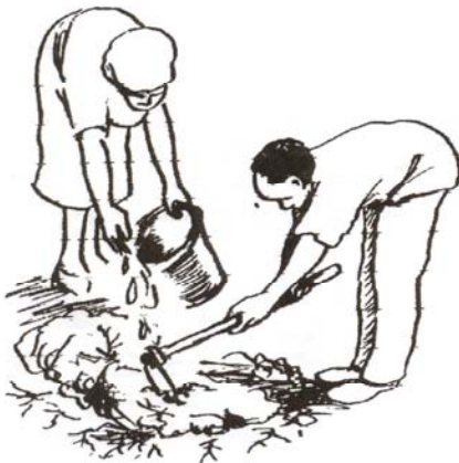
Figure 5.58 Mixing mud with water
