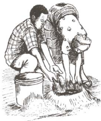
Figure 5.36 Mixing clay and sand with water
