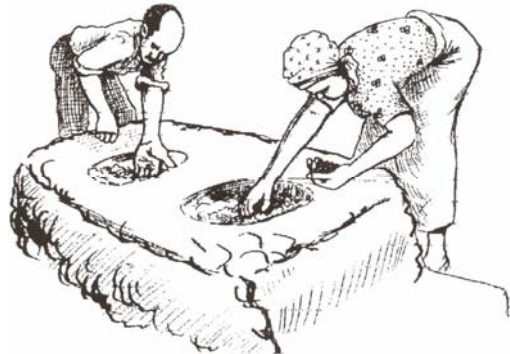
Figure 5.29 Scooping out mud to create fire chambers
