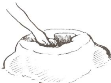
Figure 5.65 Cutting the smoke path
