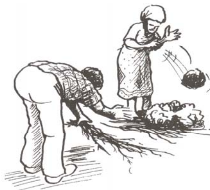
Figure 5.37 Spreading grass and throwing mud balls
