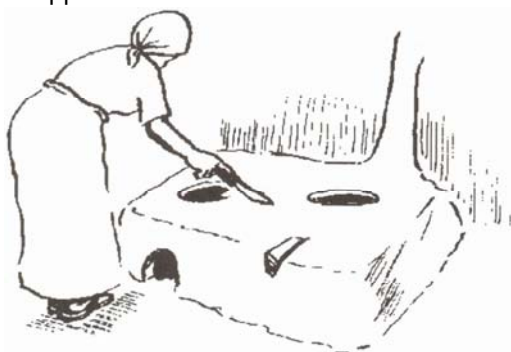
Figure A2.2 Cutting the cracked area with a knife
