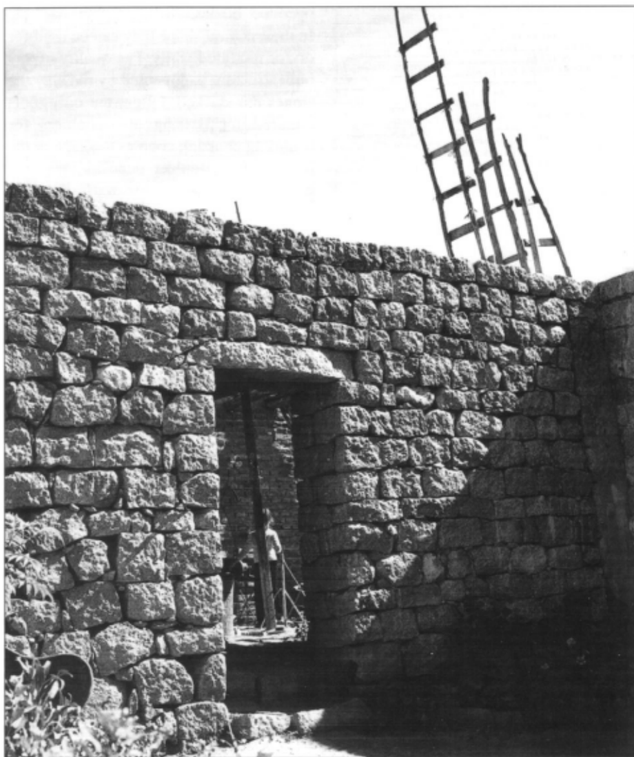
Figure 6: "Dry-wall construction with squared granite boulders in Argentina"
