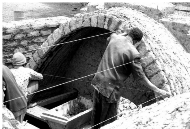
Figure 5: Guiding strings help builders maintain the alignment of the vaults.
