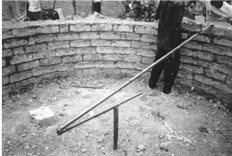
Figure 2: A mobile rotating guide at work.
