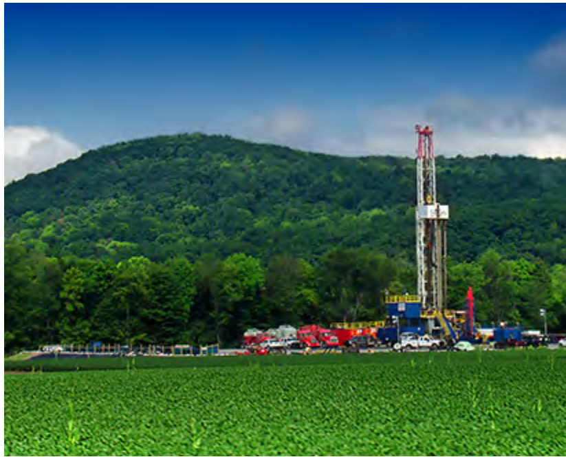
Figure 20.2 This is a Marcellus shale gas-drilling site in Lycoming County, Pennsylvania. (Photo courtesy of Nicholas A. Tonelli/flickr)
