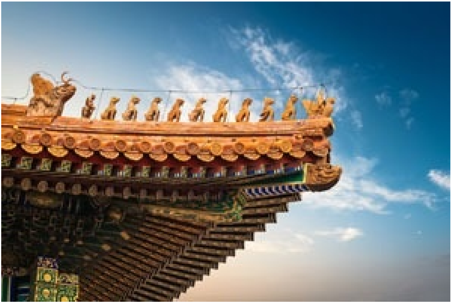
The Hall of Supreme Harmony has 12 roof ridge statuettes — left to right: an ordinary dragon head decoration, 'Series Ten' (行什, unique to this roof, an anti-thunder monkey god), then the nine animals, and a fairy decoration.
