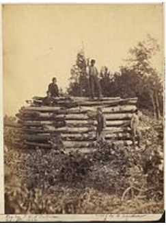
Elk Mountain (Maryland) signal tower, 1862
