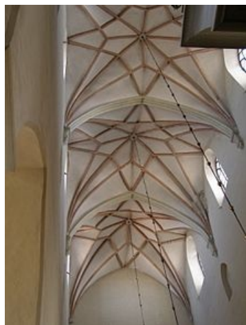
15th-century "star" rib vaults in St. Olaf's Church, Tallinn
