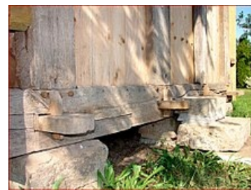
Through-wedged tenons used on a French granary.
