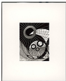
Patterns made by steel liners for diversion tunnels, Ft. Peck Dam, Montana, 1936
