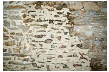
A stone wall in France with lime mortar grouting being applied. Right - unapplied, Centre - lime mortar applied with a trowel, Left - lime mortar applied and then brushed with a wire brush.
