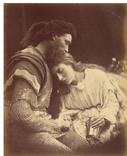
Parting of Sir Lancelot and Queen Guinevere 1874
