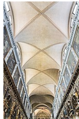
Renaissance groin vault in the church of Santa Maria dei Carmini in Venice.
