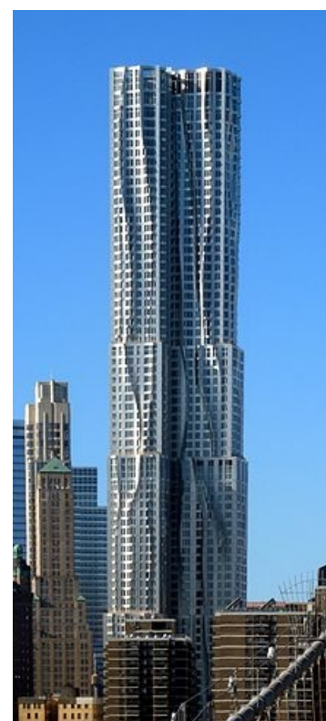
The tower at 8 Spruce Street in Lower Manhattan, completed in February 2011, has a stainless steel and glass exterior and is 76 stories high (2011)
