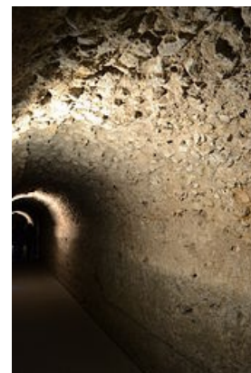
Opus caementicium exposed in a characteristic Roman arch. In contrast to modern concrete structures, the concrete used in Roman buildings was usually covered with brick or stone.
