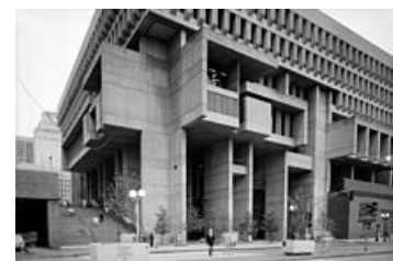
Boston City Hall (1968) is a Brutalist design constructed largely of precast and poured in place concrete. It was voted "The World's Ugliest Building" in 2008
