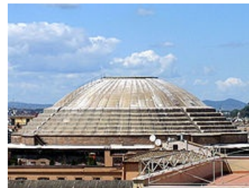
Exterior of the Roman Pantheon, finished 128 AD, the largest unreinforced concrete dome in the world. [1]
