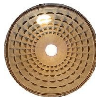
Interior of the Pantheon dome, seen from beneath. The concrete for the coffered dome was laid on moulds, mounted on temporary scaffolding.
