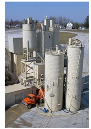
Concrete plant showing a concrete mixer being filled from ingredient silos
