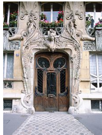
Ceramic facade decoration of Lavirotte Building by Alexandre Bigot , Paris (1901)
