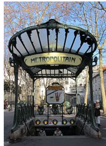
Paris metro station entrance at Abbesses designed by Hector Guimard for the 1900 Exposition universelle
