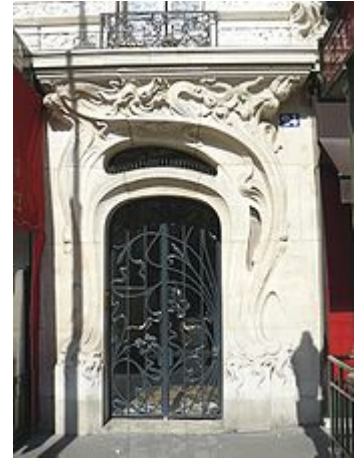
Doorway at 24 place Etienne Pernet, (Paris 15e), 1905 Alfred Wagon, architect.
