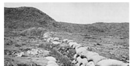
The Boer trench at the Battle of Magersfontein contributed to the surprise defeat of the Highland Brigade on 11 December 1899 during the Second Boer War.
