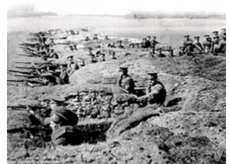
Soldiers training in trench warfare, with well-defined fire bays connected by offset traverse trenches, with zigzag communication trenches leading to the rear area
