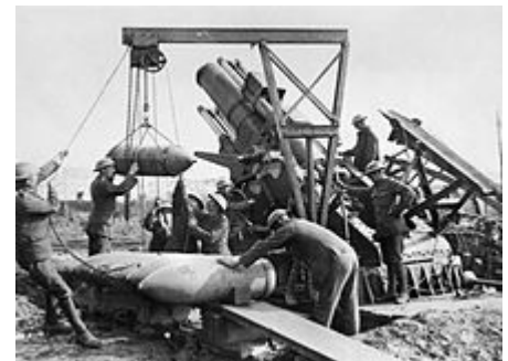
Loading a 15 in (380 mm) howitzer
