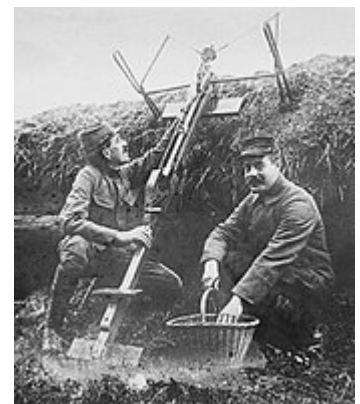
French soldiers with a Sauterelle bomb-throwing crossbow, c. 1915
