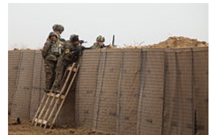
Afghan and U.S. soldiers provide security while standing behind a blast wall made from HESCO bastions at Zhari district, Kandahar Province, Afghanistan, 2012.
