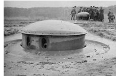
A retractable turret of Ouvrage Hochwald, one of the largest fortifications of the Maginot Line, 1940
