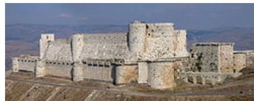
Krak des Chevaliers was built in the County of Tripoli by the Knights Hospitaller during the Crusades.
