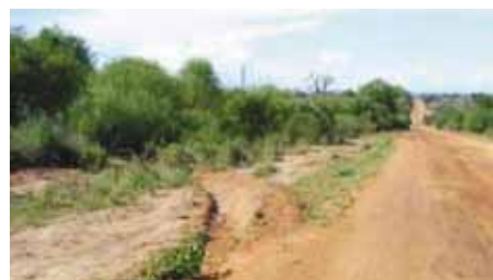
Run-off water from roads can be harvested from cut-off trenches or road ditches
