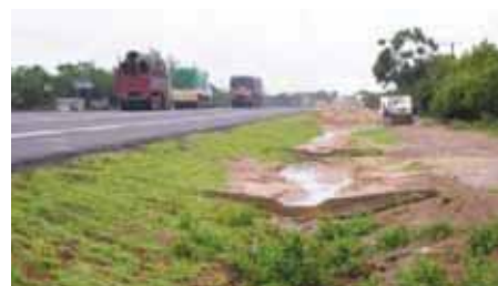
Run-off water from roads can be harvested from cut-off trenches or road ditches
