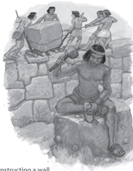
Constructing a wall
